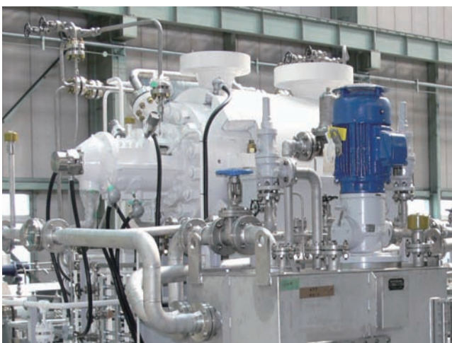
Saudi Kayan Petrochemical Complex Saudi Arabia MHB, Boiler feed water pump
