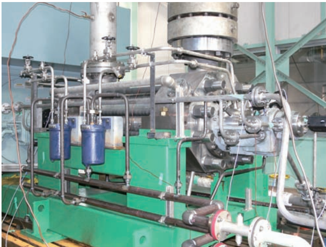
Emal Aluminum Smelter Complex UAE MHG, HP Feedwater pump
