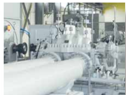
Water Transfer Pump for Shuquaiq II Abha Pump Station (Saudi Arabia) Pump type: MSH300/2T, Delivery year: 2009 Duty: 2,325m 3 /h at 722m, Power: 6,150kW
